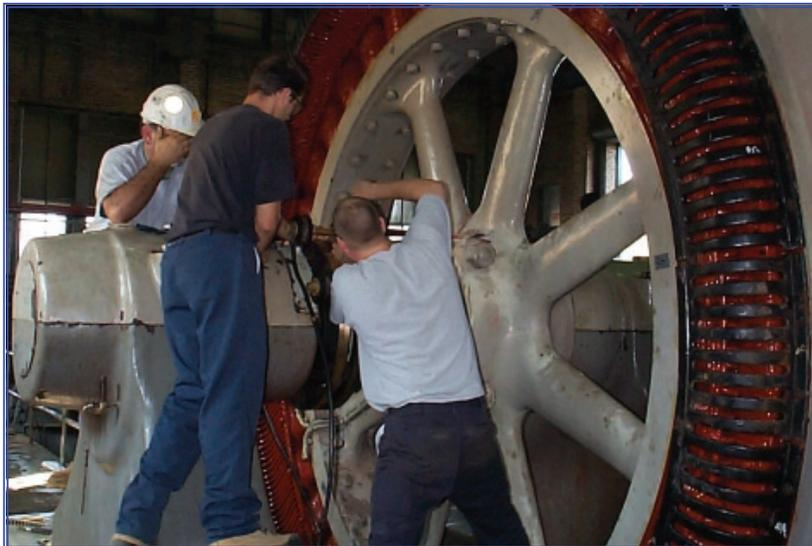
Flood waters from Hurricane Katrina submerged many of the giant motors which power the massive pumps of the S&WB's Drainage System. Within three days of the storm's passing, the Board had arranged for a team of experts from the General Electric Corporation to come to the City to work with S&WB staff to dry the motors and begin the re-winding process.
