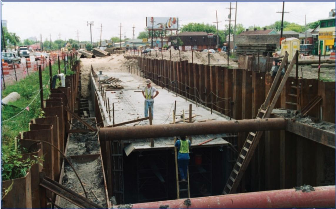
A new concrete subsurface box canal beneath South Claiborne Avenue is just one of many SELA projects completed, underway or in the design stage.
