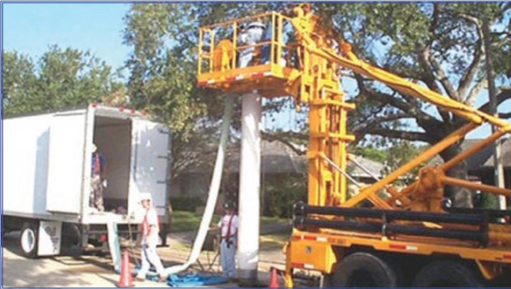
SSERP uses trenchless “no dig” techniques whenever possible to repair sewer lines. Here, a polyester felt liner is inserted inside a damaged pipe, then cured in place with hot water to the shape of the broken pipe. The lining system fills breaks in the line without needing to dig into the street at every break in the line.
