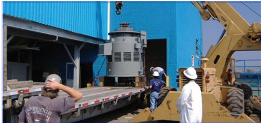
It was crucial to dry out and repair generators, motors and wiring quickly before salt water destroyed them. Crews were working on the day after the storm passed.
