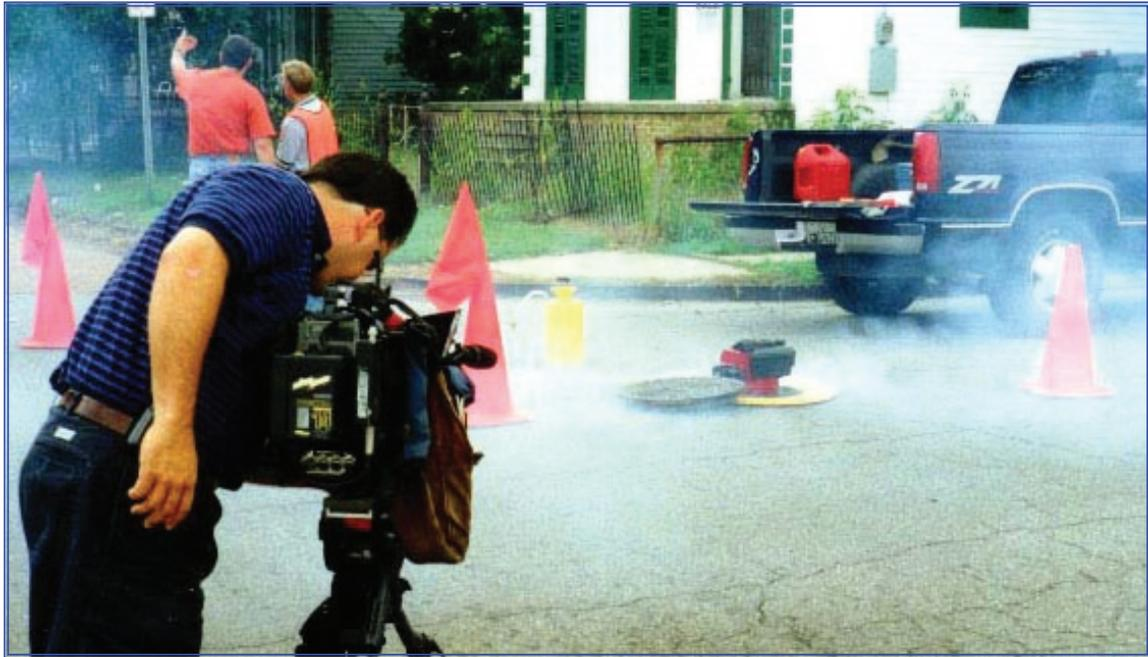
Smoke testing is one of the methods used to detect leaks or breaks in sewage lines.
