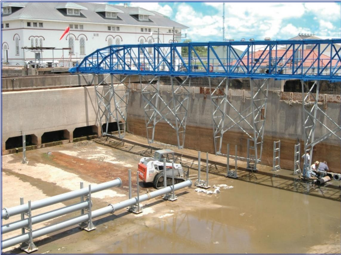
Sediment basins at the Carrollton Water Purification Plant were damaged by Katrina and are now under repair.
