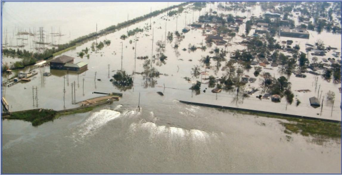
Breach in the Industrial Canal Flood Wall
