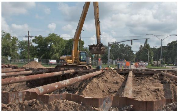
Work has begun to improve drainage in the the Gen. DeGaulle Canal in Algiers. It is a project funded by the Louisiana Department of Transportation and Development. The entire Algiers Area Drainage Improvements program is being evaluated by the Corps of Engineers for inclusion in the federallyfunded Southeast Louisiana Urban Flood Control Project.
