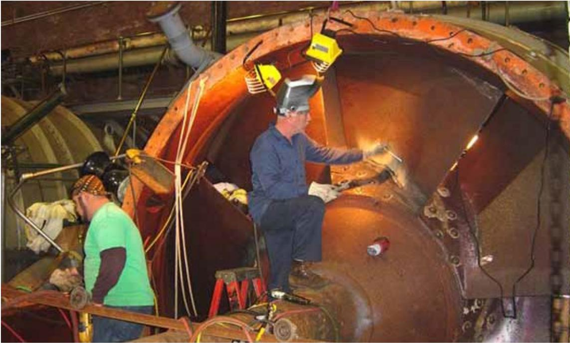
When one of the pumps at Drainage Pumping Station No. 3 began to “chatter” and make a loud noise, it was discovered that 5 of the 8 impeller blades were cracked. The Board’s own employees from Facility Maintenance disassembled the pump, gouged out the cracked areas and weld-repaired the blades.
