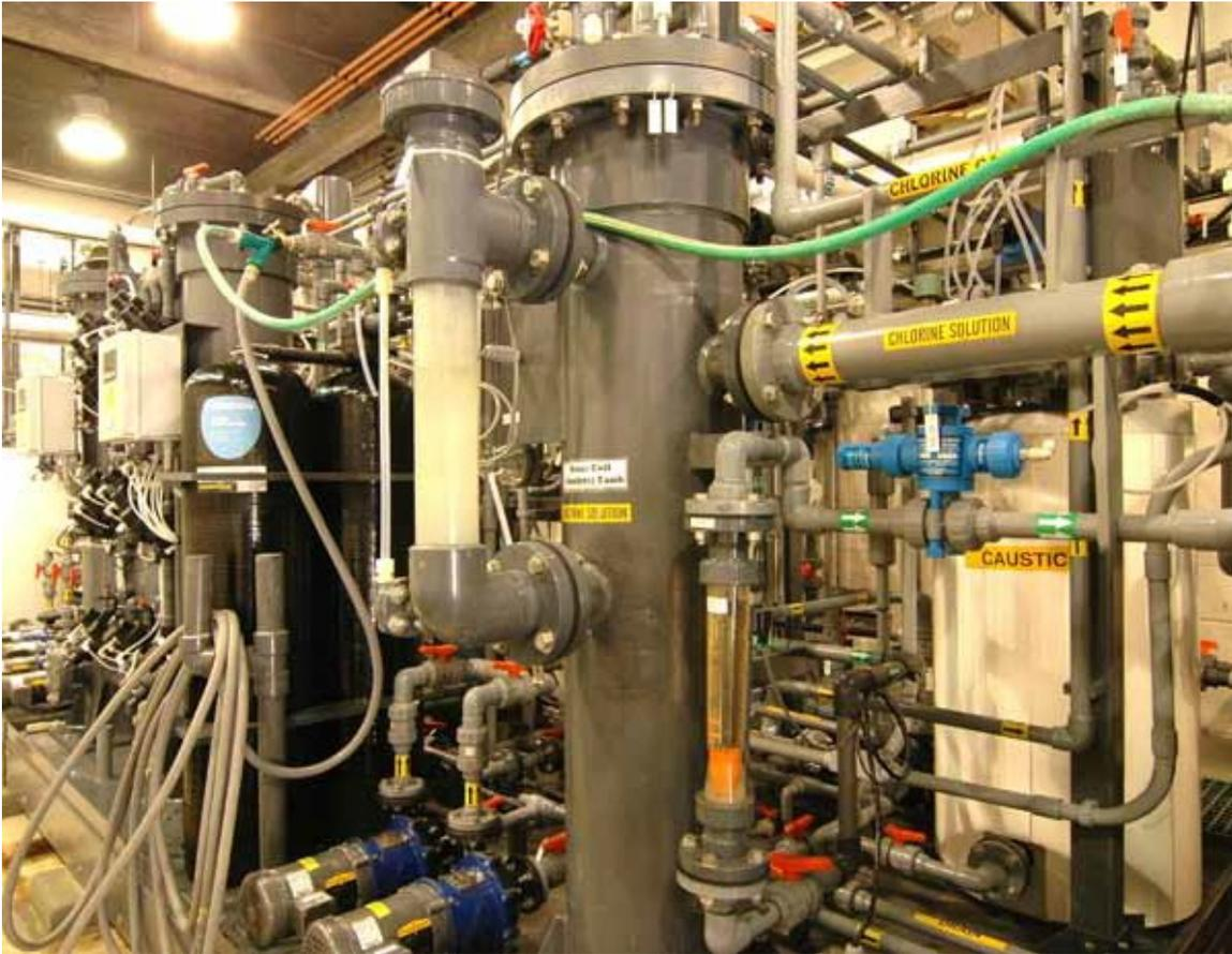
A new \$2 million Klorigen Unit is now in operation at the Algiers Water Treatment Plant. The unit produces chlorine disinfectant on demand for the water treatment process by using food-grade salt and electricity. The driving force for using this system is risk reduction by eliminating the need to store tons of liquid chlorine onsite which could release to the atmosphere.
