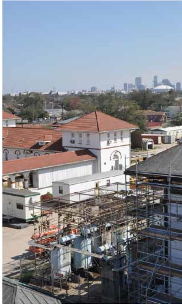
The Sewerage & Water Board's staff is constantly developing and exploring new processes to improve its operations. One such project is underway at the Carrollton Water Purification Plant. The Sodium Hypochlorite Bulk Storage/Feed Facility is set for completion in 2012. It will eliminate the need for transporting chlorine by rail and storing it on the plant grounds. Instead, the Board will use the safer
